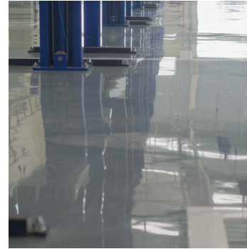
Epoxy and PU anti-static flooring
